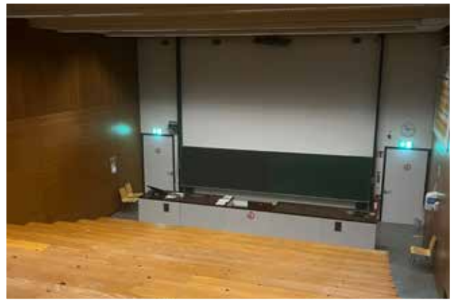
Martin Luther King Square 6 "Very old lecture halls with poor acoustics, no windows....In addition, in the corridors for some time are very large holes in the ceilings under which there are buckets. The laboratories are also outdated, as they have not been renewed since they were built."
