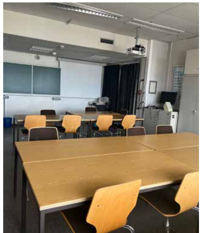
Geomatics Room 1643 “very loud heating/ ventilation and leaky door”
