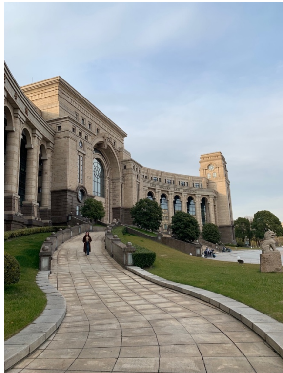
Picture 8: Building of the Law Faculty on Jiangwan Campus
